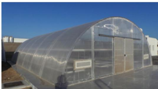
**Fig. 1.** Polycarbonate Drying House (PDH)
